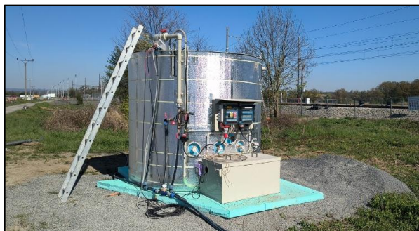
Obr. 4 a 5 Bioreaktor pro aplikaci biodegradace in situ a isokontejner na \text{H}_2\text{O}_2 pro chemickou oxidaci ISCO Fig. 4 and 5 Bioreactor for in situ biodegradation application and \text{H}_2\text{O}_2 isocontainer for chemical oxidation ISCO
